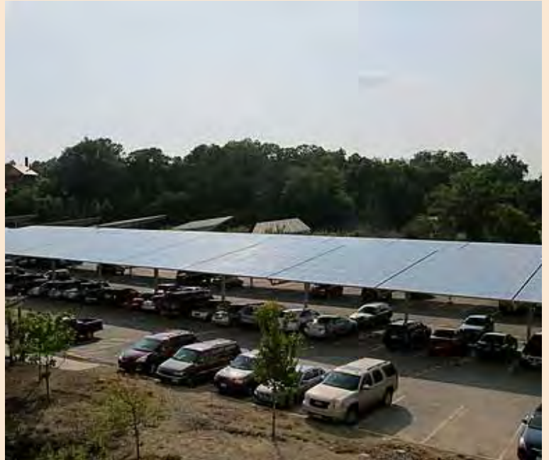
Solar canopies at the Cincinnati Zoo generate 1.6 MW of energy
